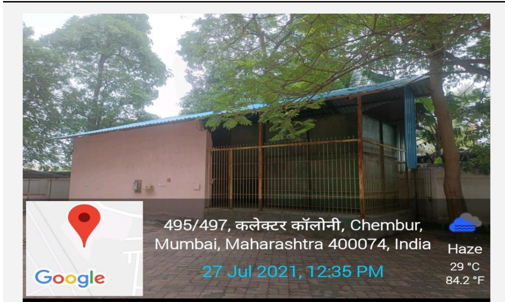
Figure- Sewage Treatment Plan (Image 1)
