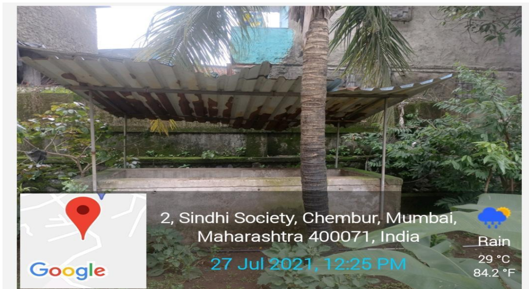
Figure- Compost pit installation at VESIT (Front view)
