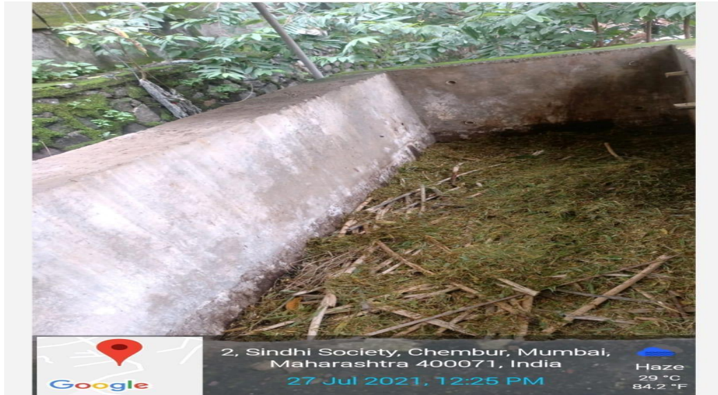
Figure- Compost pit installation at VESIT
